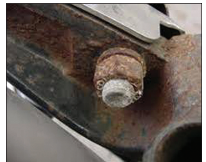
Figure 11. Rusty Bolts can cause PIM.
