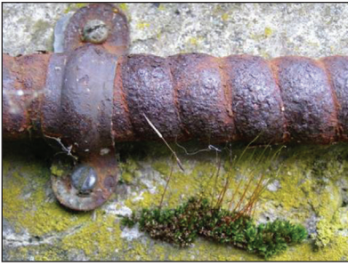
Figure 29. Cleaning up sources of PIM can cure interference problems.
